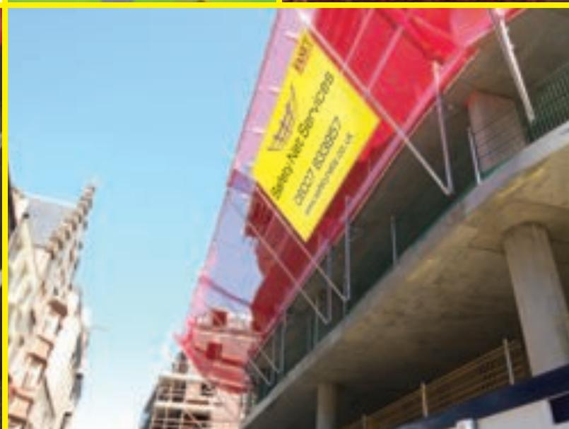
“SAFETY NET SERVICES HAVE DEVELOPED A UNIQUE SYSTEM FOR RAISING & FITTING SAFETY NET FANS WITHOUT THE NEED TO RELY ON THE USE OF A TOWER CRANE. THIS ENSURES THE FANS ARE INSTALLED IN A SAFE AND EFFICIENT MANNER WITH MINIMUM DISRUPTION TO OTHER TRADES.”
