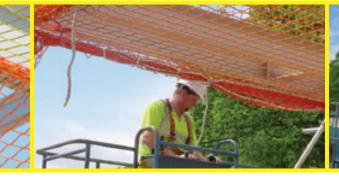
The modern, lightweight safety nets used by Safety Net Services are fitted as close to the work position as possible. By fitting safety nets so close to the working level they prevent a fall causing personnel injury and also offer a collective level of protection, as such, they are an improvement on the use of harnesses and lanyards.
