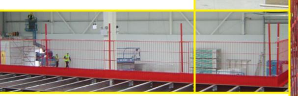
The steel mesh barrier is simple to join, is very robust and has a built in toe board, which is standard requirements today and can be fitted into a wide range of attachments, selected according to the constructional situation.
