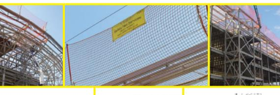
Prior to any installation we can produce design sketches and calculations to prove system integrity, if installed with the safety nets it will provide total encapsulation and provide an element of debris containment.
