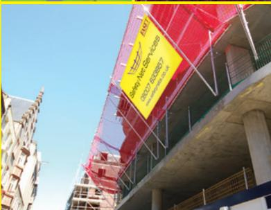
\*\*SAFETY NET SERVICES HAVE DEVELOPED A UNIQUE SYSTEM FOR RAISING & FITTING SAFETY NET FANS WITHOUT THE NEED TO RELY ON THE USE OF A TOWER CRANE. THIS ENSURES THE FANS ARE INSTALLED IN A SAFE AND EFFICIENT MANNER WITH MINIMUM DISRUPTION TO OTHER TRADES. \*\*\*
